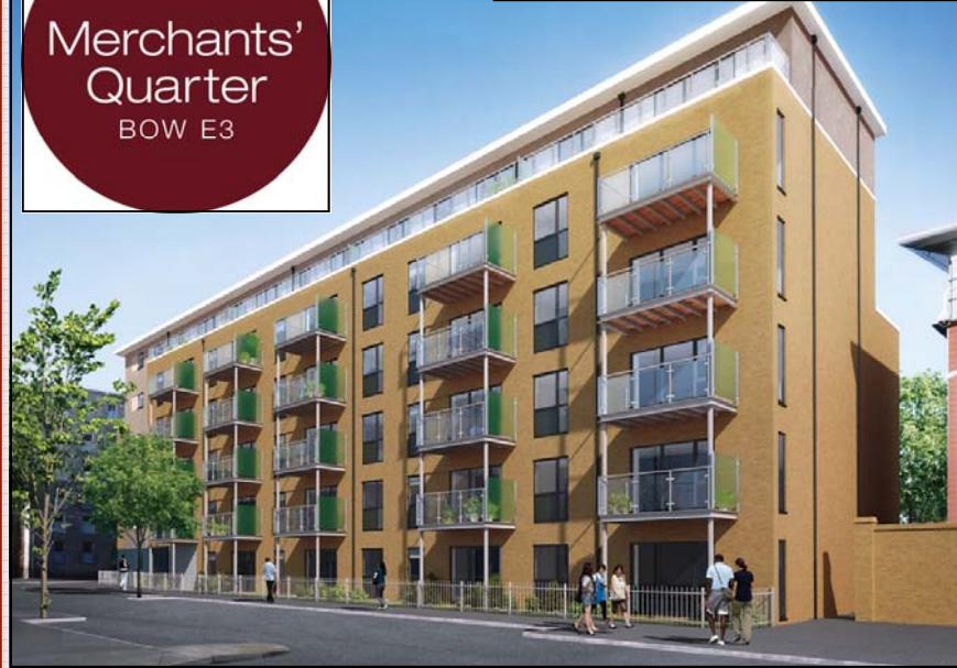
Latest computer generated image of Saunders Apartments from Merchant Street.
